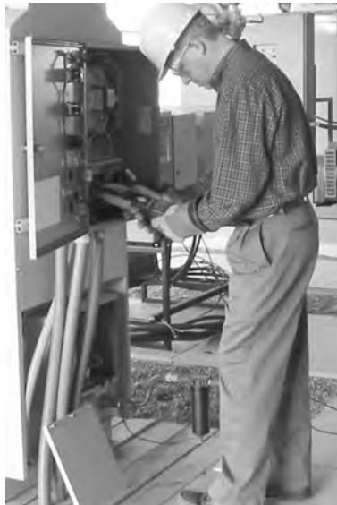
Figure 5-1—Power line monitor
